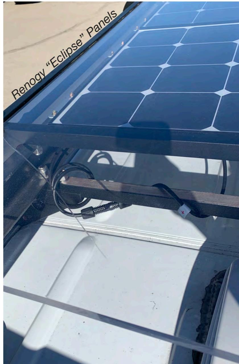
On the roof, (4) 100-amp solar panels are connected in series. Series, not parallel because Renogy Eclipse panels have bypass diodes, which allow current to flow, even in partial-shade condition.
