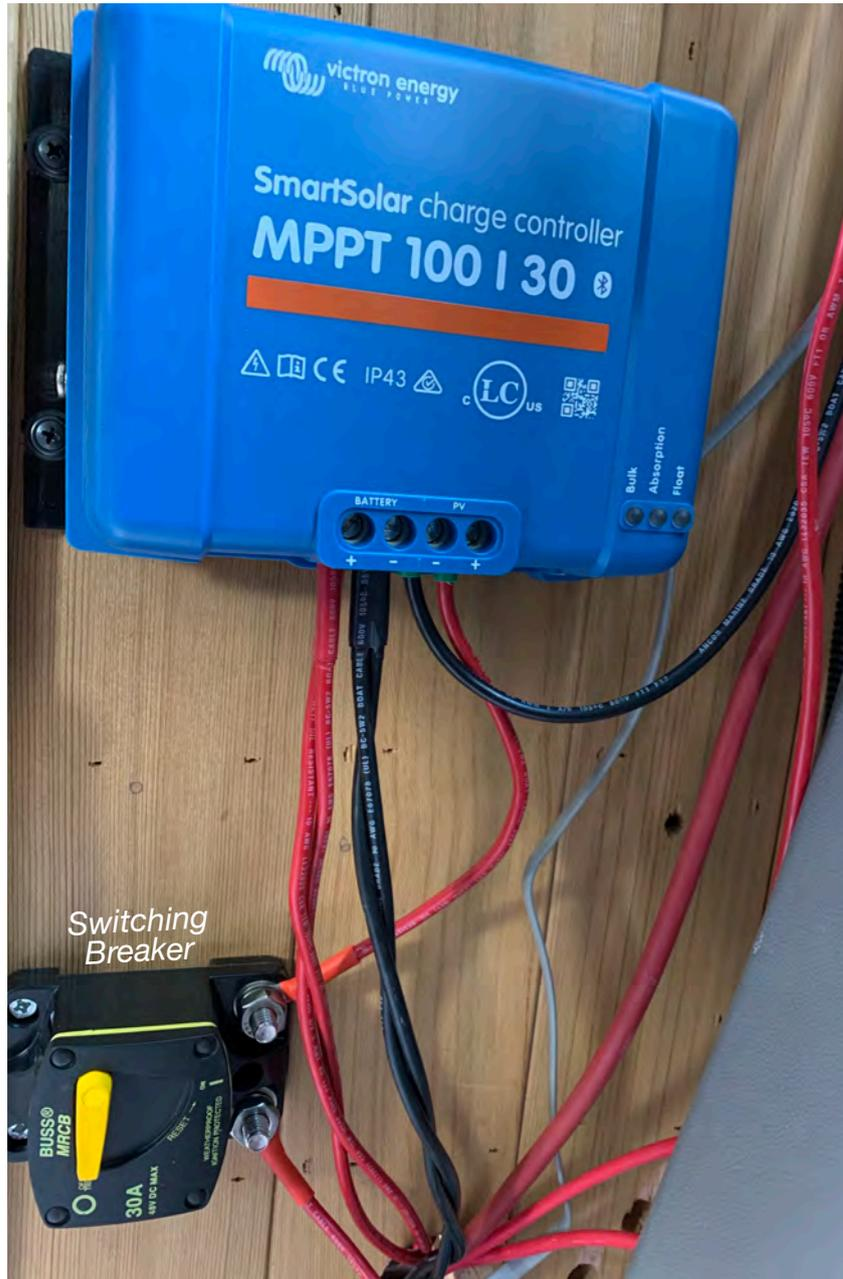
Solar controller on outside of sofa bed, directly behind driver's seat. The black and yellow breaker isolates panels from controller. Deliberately, there is NO switch between controller and battery.
